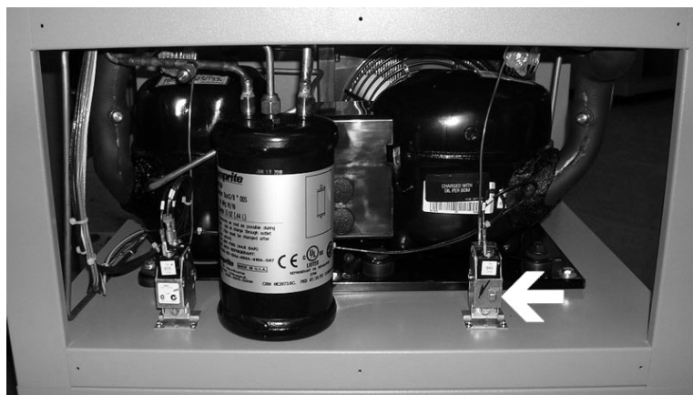
Figure 8-1 – PS2 Pressure Switch Reset Button (lower rear panel removed)
